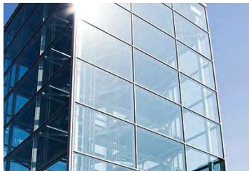
F13: CAR PARK FACADE
