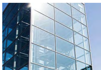
F13: CAR PARK FACADE
