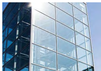
F13: CAR PARK FACADE
