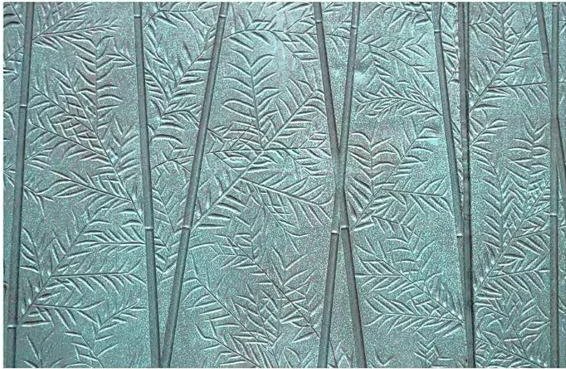
STENCILED PRE-CAST CONCRETE PANELS
