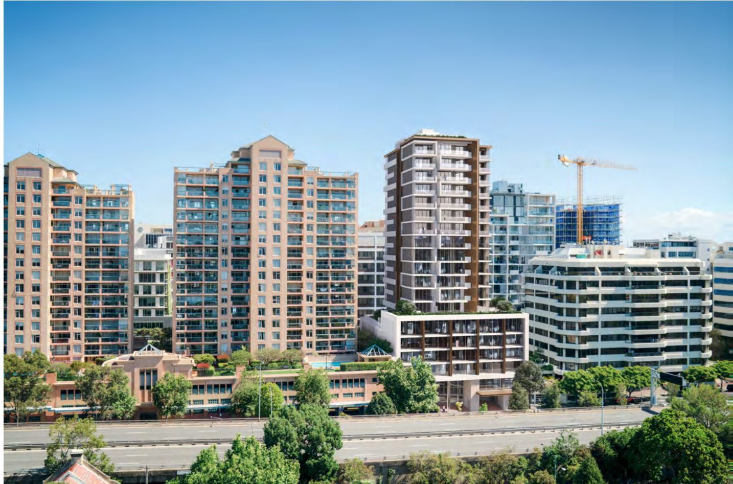
AERIAL VIEW FROM NORTH EAST - APPROVED DA
