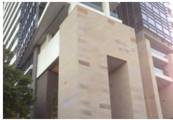
F1: SANDSTONE CLADDING MIN THICKNESS 30MM
