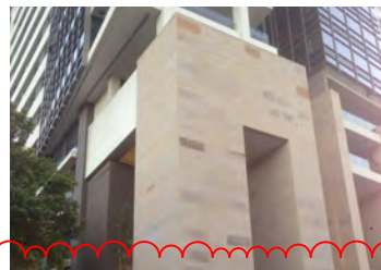
F1: SANDSTONE CLADDING MIN THICKNESS 30MM
