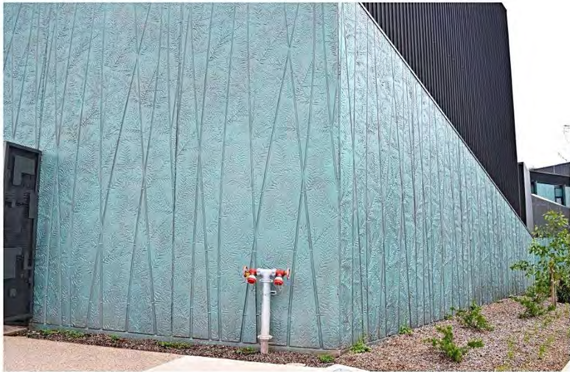
STENCILED PRE-CAST CONCRETE PANELS
