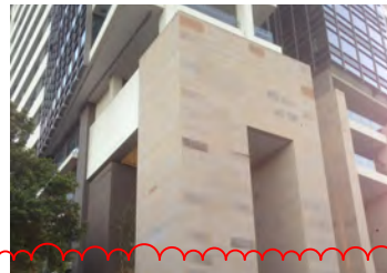
F1: SANDSTONE CLADDING MIN THICKNESS 30MM
