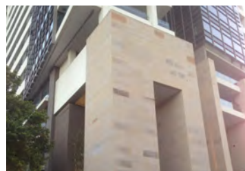
F1: SANDSTONE CLADDING MIN THICKNESS 30MM
